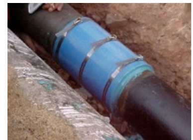
EXTERNAL CORROSION REPAIR
