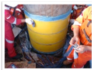
OFFSHORE CAISSON LEAK REPAIR
